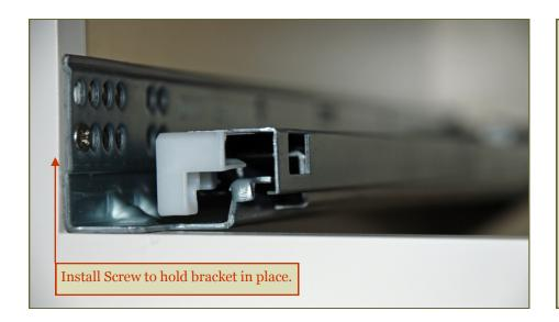
Insert / connect glide assembly over plastic boot in back of cabinet.
