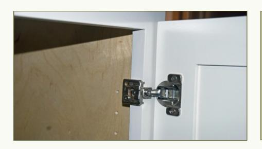
Fasten Hinge Cup to the door with screws furnished. The hinge will then be fastened to the Frame.
