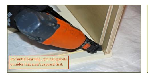
Drop side panel into the face frame dado and lightly tap top of the panel with mallet to solidly seat panel into dado.
