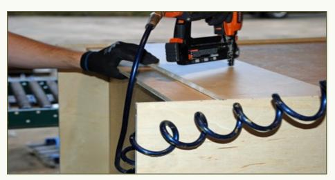
The Hanging rails are fastened on the back of the cabinet. Top rail is flush with the top of the back panel. Bottom rail should be positioned approx. to bottom of the floor on (base) and flush with the bottom of the back panel on wall cabinets. These should be glued and pinned.
